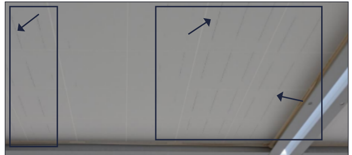
Backsheet failure in the field
