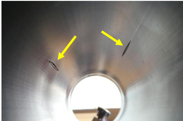
Figure 6. Pipe failure after testing in the horizontal container. Two cracks are visible at the top of the pipe (yellow arrows), although only one has failed.
